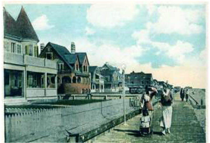
Bay Head Boardwalk, looking north from Bridge Ave., C.1935
